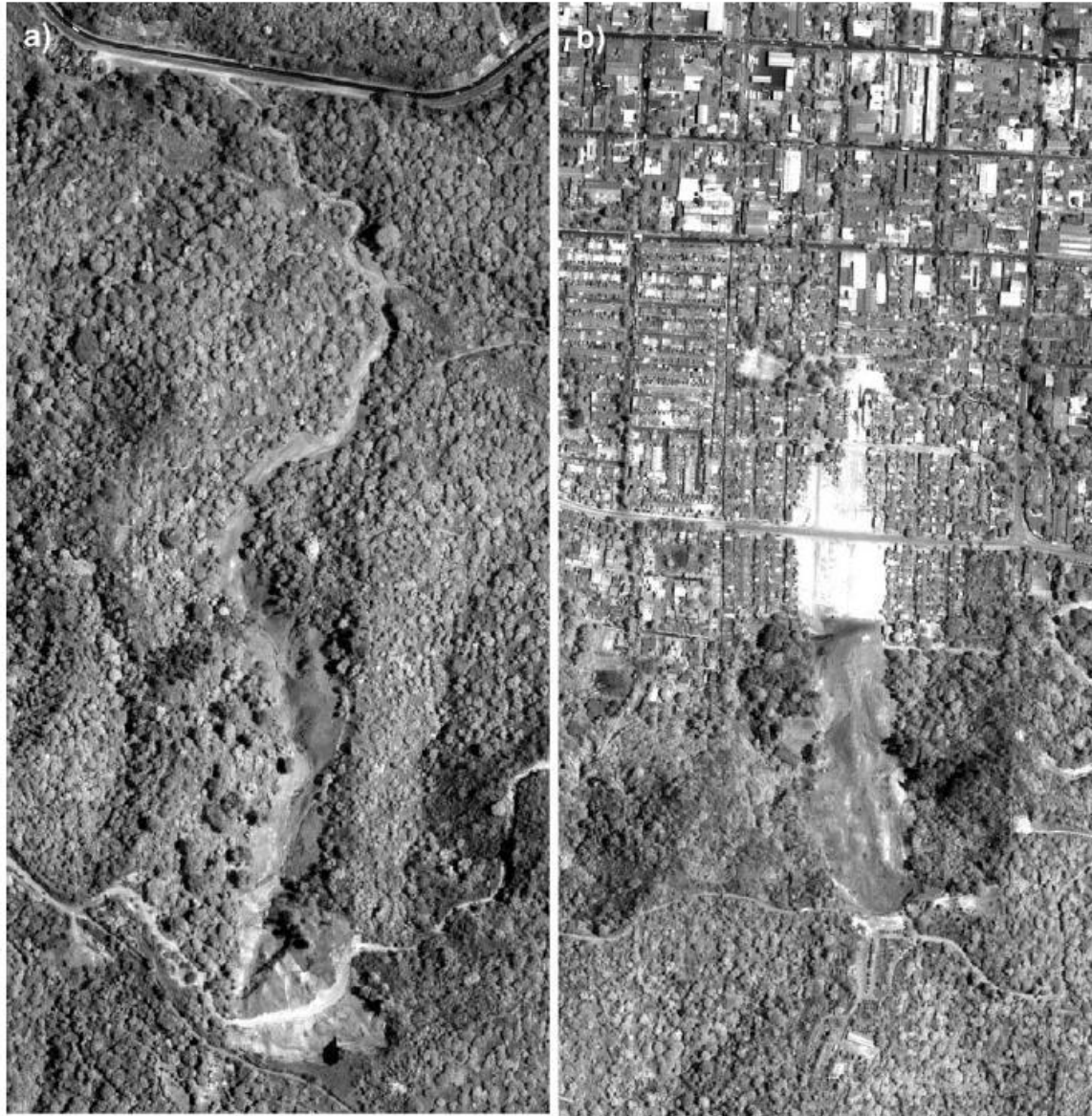
Fig. 3. (a) Las Barrioleras Landslide, SW of the Nueva San Salvador and few kilometers to the W of the (b) Las Colinas landslide. Photos are at the same scale.
